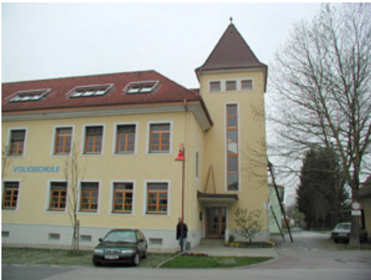
SCHOOL MARKT HARTMANNSDORF
